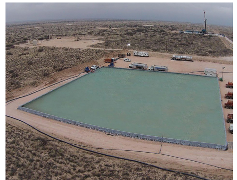
Primary & Secondary Containment
