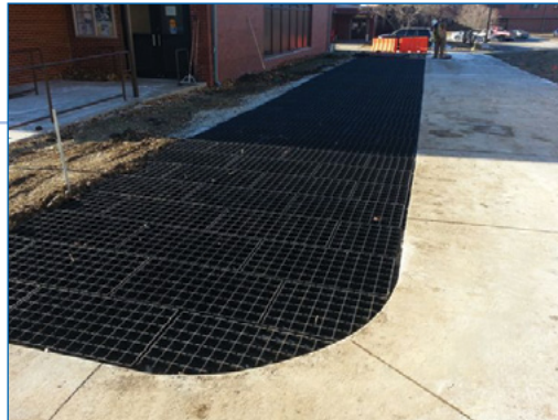
4 Geoblock is easily cut with a reciprocating saw for curved edges.
