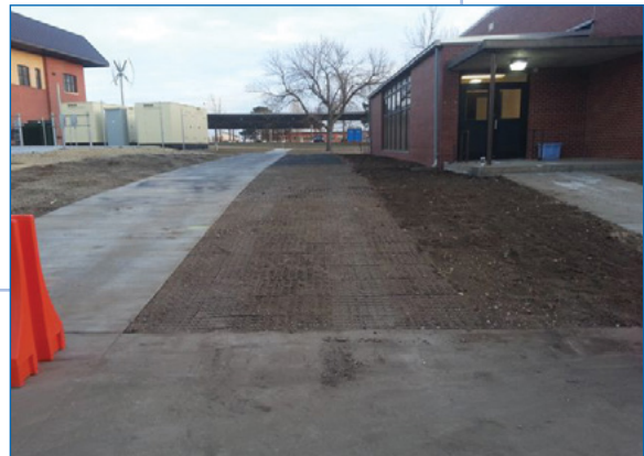
6 The area was seeded early spring 2014. Blueville Nursery also chose to cover the new seed with hydromulch knowing that the area was not irrigated.
