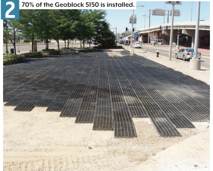
2 70% of the Geoblock 5150 is installed.
