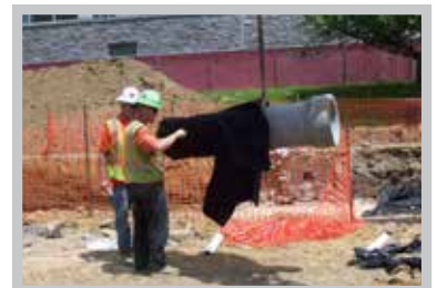
Fig. 16 Seal the pipe boot with the included band clamps and duct tape.
