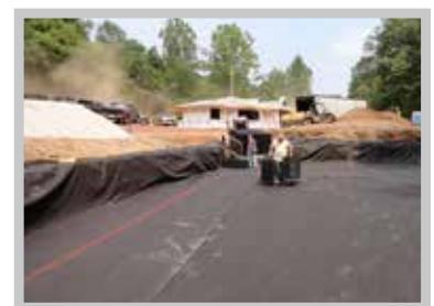
Fig. 5 Use a string line and marking paint to square the system footprint.
