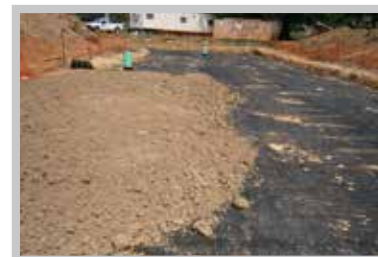
Fig. 20 Pushing backfill parallel to the Geogrid prevents the grid from shoving.
