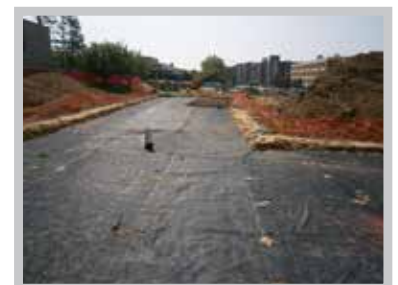
Fig. 19 Overlap Geogrid 18" or as required by plans.
