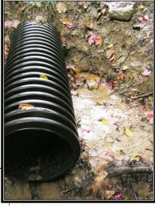
(Above) Water "piping" on the <u>outside</u> of a corrugated pipe following the annular space in the trench (preventable with an anti-seep plug of AquaBlok)
