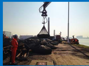
Belgium 2014 scour protection
