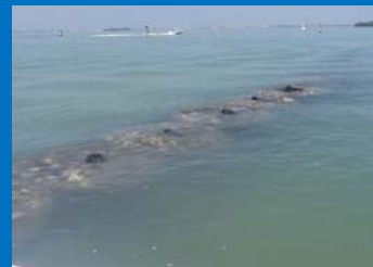
Italy 2009 create canal dike
