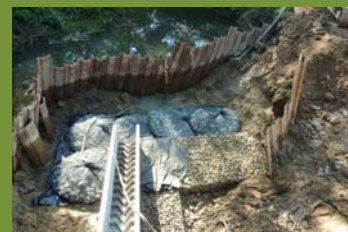
U.K. 2014 foot protection with gabion
