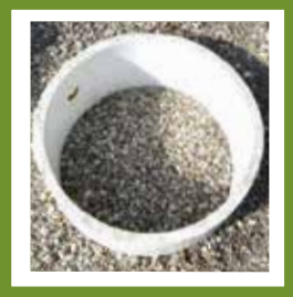
Figure 4: Pipe Installed Into Media
