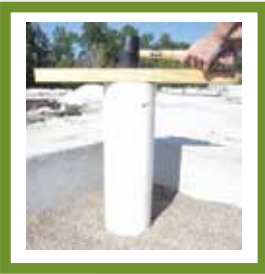
Figure 3: Hammering Pipe Into Media
