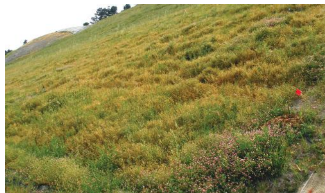
A well planned erosion control solution tailored to your site can eliminate costly reconstruction of degraded slopes.
