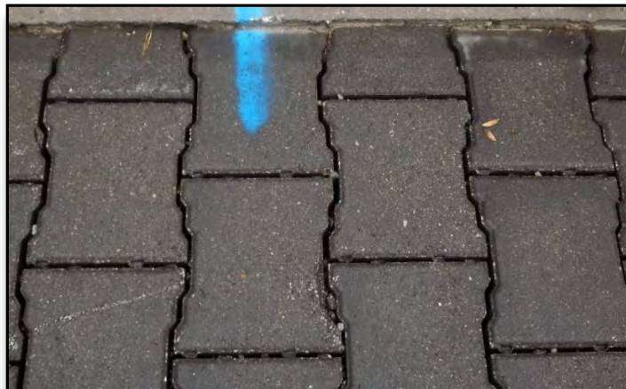
Photo 2 – PaveDrain following maintenance
