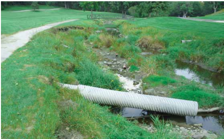
stream banks & toe of slope
