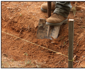
1. Stake out/remove sod
