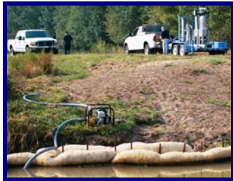
Turbid water is first treated with BIOSTAR™ CH, then sand filtered
