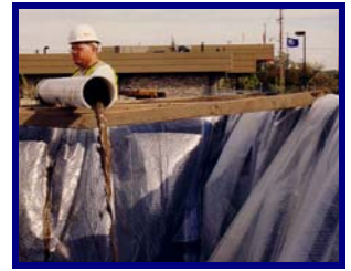
1. Dewatering using temporary storage
