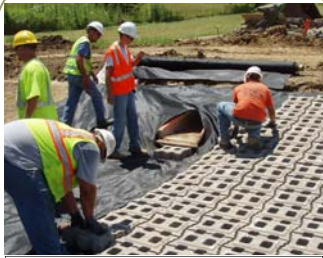
Workers hand placing the UltraFlex articulating concrete blocks in line.
