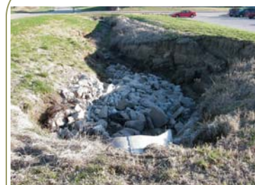
This is what the swale looked like before installation.
