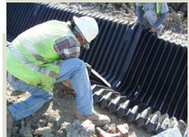
The joining of two sections
