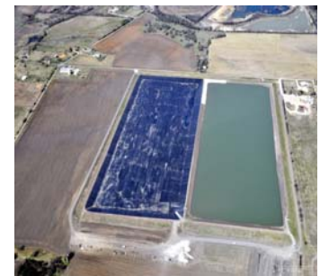
Waste Water Treatment Plant
