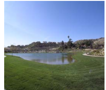
Stormwater Treatment Pond
