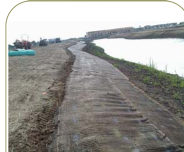
Installation of the Vmax3 C-350 Turf Reinforcement Mat
