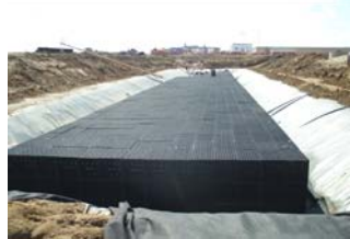
1,079 Triples Atlantis D-Raintanks were assembled and placed on the a 6" sand layer on liner bottom.
