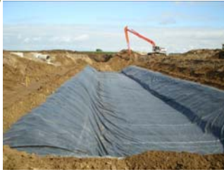
The excavation was completed and the fabric and liner was installed.
