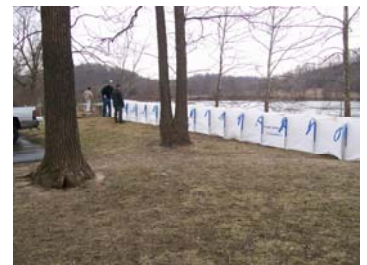
Completed Installation- property protected!!
