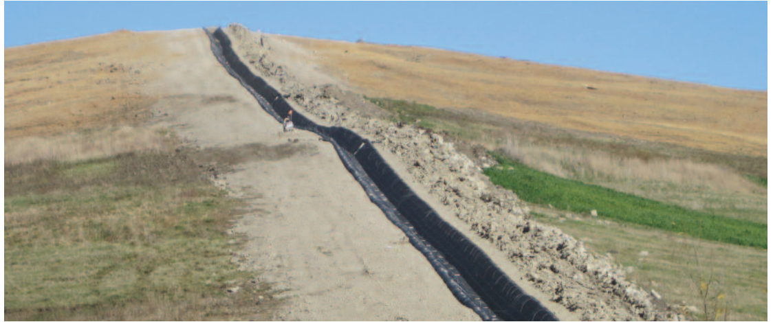
2,750 feet of 24" Trapezoidal SmartDitch Liner was used to control erosion and stabilize slopes at the Newton County, Indiana Landfill. SmartDitch's proven water flow control characteristics, low maintenance and ease of installation made it the best option for this project. The bulk of this installation took just 3 days and a crew of 5.
