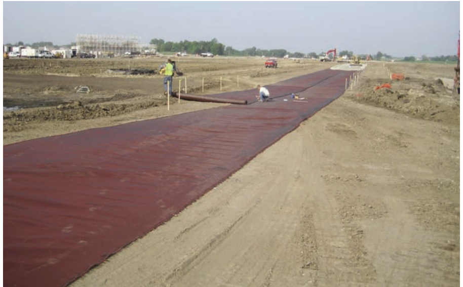
Mirafi® RS580i being installed over weak subgrade.
