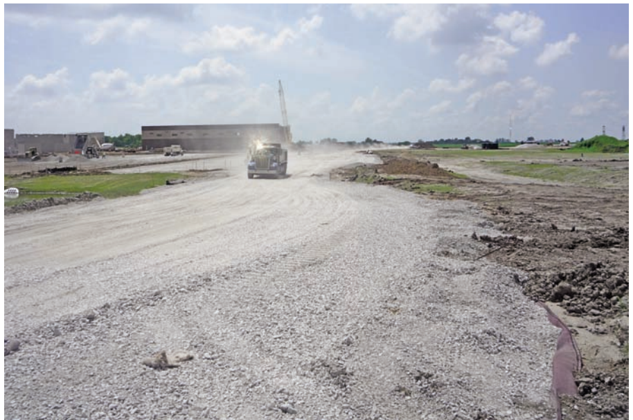
Installation complete with 6" aggregate.
