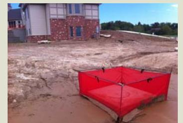
Over 3 acres of disturbed land drain into this area inlet. Note the sediment build up.
