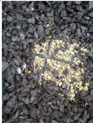
The Geopave was in-filled with angular stone and then surface treated with a decorative mulch.
