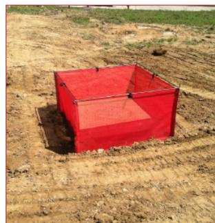
"Big Red" AI Protector, recently installed with trenched in bottom and tight sides.
