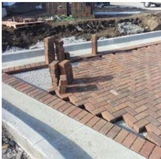
A concrete curbing was used to edge the pavers.
