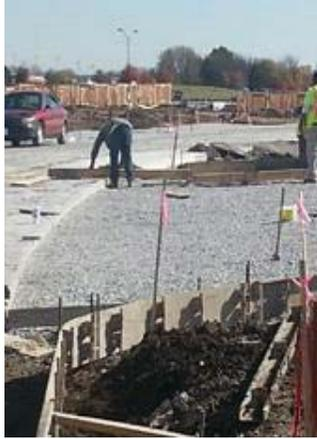
Pavers installed on 12" of clean rock for water storage.
