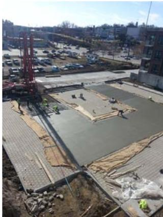
Once the PaveDrain was installed, the concrete was then poured in the remaining areas.
