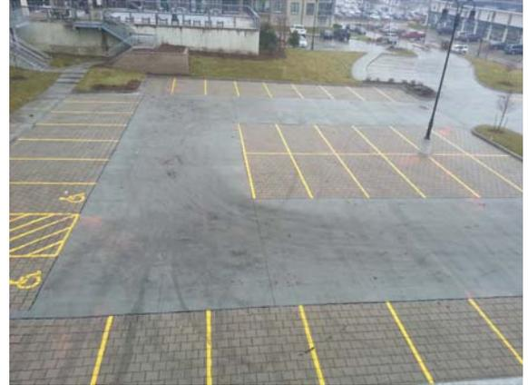
**Project Scope:** Through the help of grant money to support their efforts, permeable pavement was wanted for this parking lot. Several paver systems were reviewed and PaveDrain was utilized because of its ease of installation, being cabled, and its strength. The engineers at Cooper decided to utilize PaveDrain for all of the parking stalls and pour concrete for the remainder of the traffic areas, mostly to keep the cost in check.
