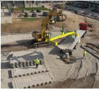
Unloading the first trucks for stockpiling before installation begins.
