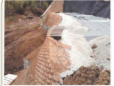
Utilizing stretcher frames, the Geoweb wall panels are placed and filled with ease.
