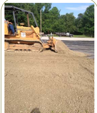
Care was taken for rock placement to not excessively wrinkle the geogrid.
