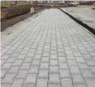
Note the sediment protection on the right. It is critical that permeable paving solutions be protected from construction sediment and debris.
