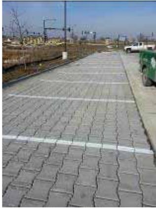
PaveDrain after installation and striped. Each block is approximately 1 square foot (nominal).
