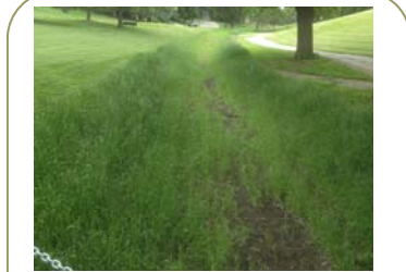
Vegetated, shear stresses can exceed 15lbs per square foot.
