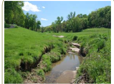
This is the channel before work began. Severe erosion is obvious.
