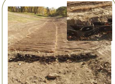
Immediately after construction, the Geoweb with C-350 on top can withstand significant forces.
