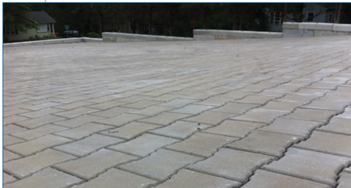
7 The finished system provides infiltration, storage, detention, conveyance and a paving surface all in one.
