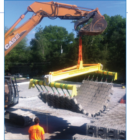
5 PaveDrain arrives on site cabled into large mats.
