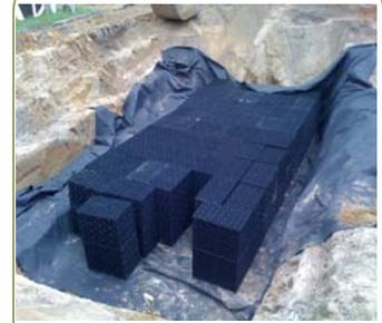
*Infiltration tanks being installed under a geotextile layer. This 2500 gallons storage volume was installed in one day with a crew of 4.*
