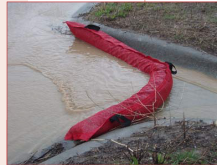
1 "Big Red" CI protector protecting a concrete swale.
