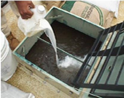
Emulsion or powder **Silt Stop**® may be added to a hydroseeder as the final additive in the mixture. Each **Silt Stop**® type may react differently in regards to the soil type that is being targeted. Specific soil tests will determine the correct **Silt Stop**® that will need to be used.
