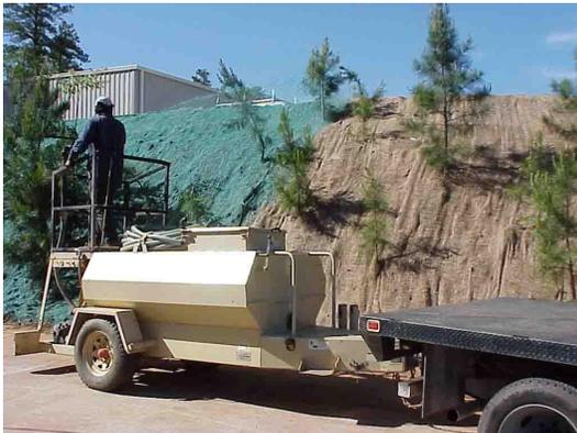
Combining **Silt Stop**<sup>®</sup> with the hydroseeding mix and applying over soft armor provides a secure base for vegetation to grow.
