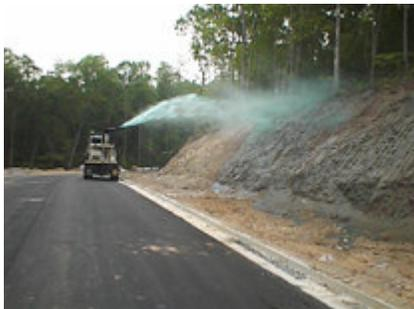
Application of the hydroseeding mix will vary with the viscosity of the solution. Different **Silt Stop**® types will create different viscosities. In most cases applicators may not see a difference in the mix solution. Conventional tackifiers need not be used when using **Silt Stop**® within your hydroseeding mix.
