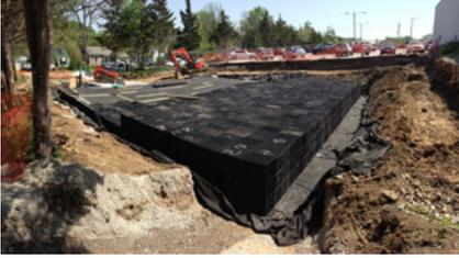
Atlantis tanks installed and ready for crushed rock placement.
