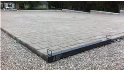
PaveDrain installation completed. ASP bump bar shown is used to tighten up all block spacing.
