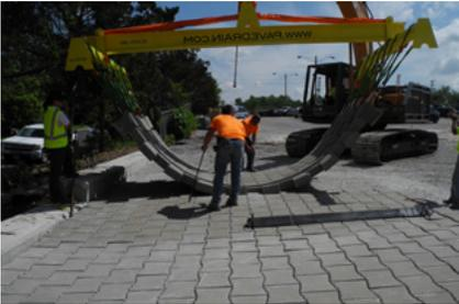
PaveDrain Spreader bar being used to place 7.5'x 17.5' panel into place.
