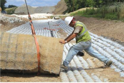
Flexamat installation with 1 track hoe operator and 1 worker in the channel.
