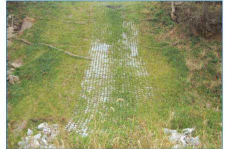
Vegetation establishing on the slope and swale.
