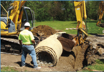
Anchor trench at the dead end.
