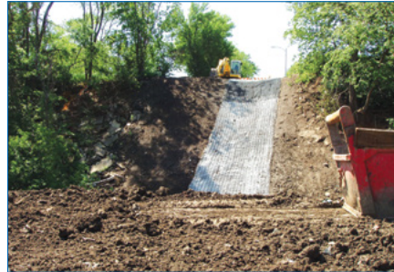
Earth anchors used only at geogrid splice area.
