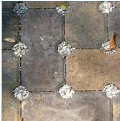
5 Close up view of how water gets through the joints of the permeable pavers.
