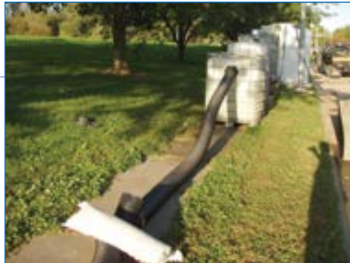
3 Gravity moves the water through the treatment train.
