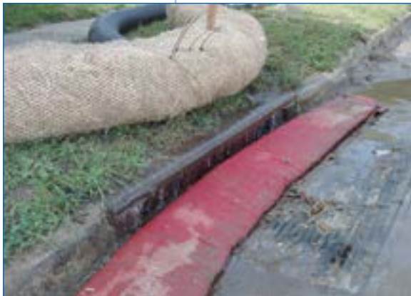
5 Excelsior Log used for final filtering.
