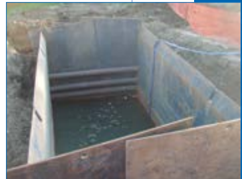
1 Pumping from the collection pit.
