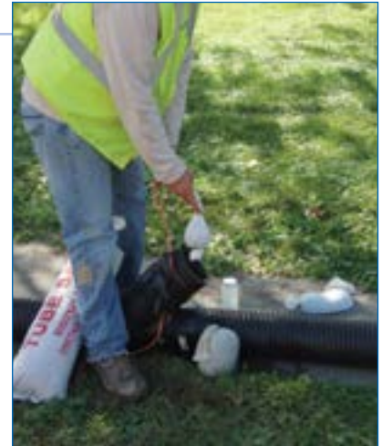
4 Floc bags tied off into the pipe.
