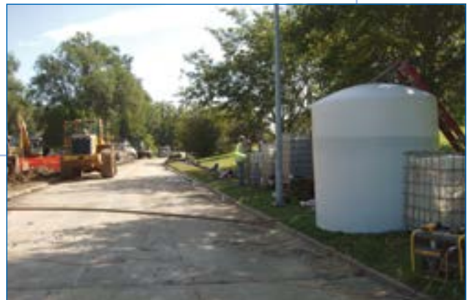
6 Limited jobsite space for other alternatives.
