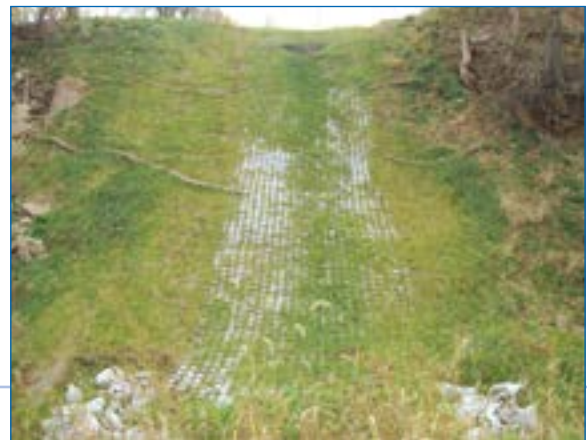
7 Vegetation establishing on the slope and swale.
