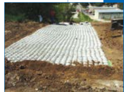
3 First mat anchored, backfilled and compacted.
