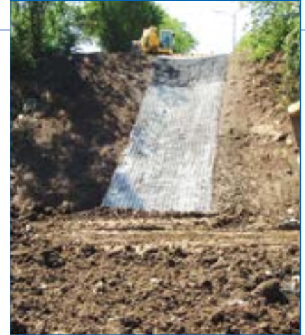
5 Earth anchors used only at geogrid splice area.
