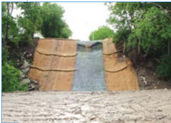
6 Coconut erosion blankets on either side of swale.
