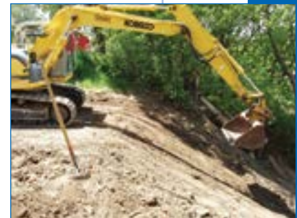
1 Grading a swale on slope face.
