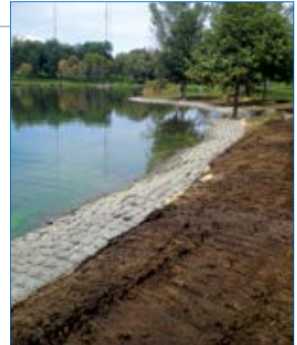
5 First day installation results.
