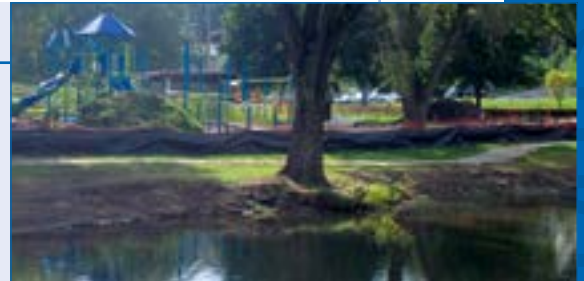
1 Sycamore tree erosion.
