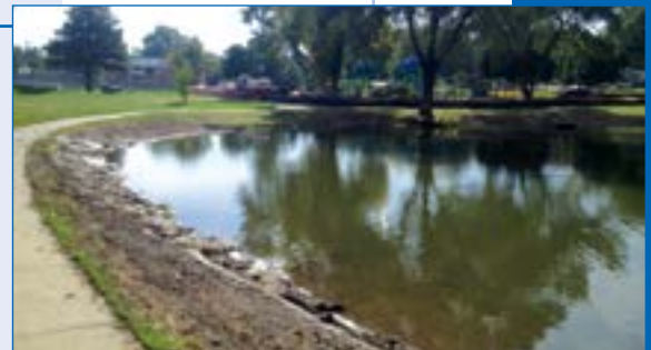
2 Shoreline before installation.
