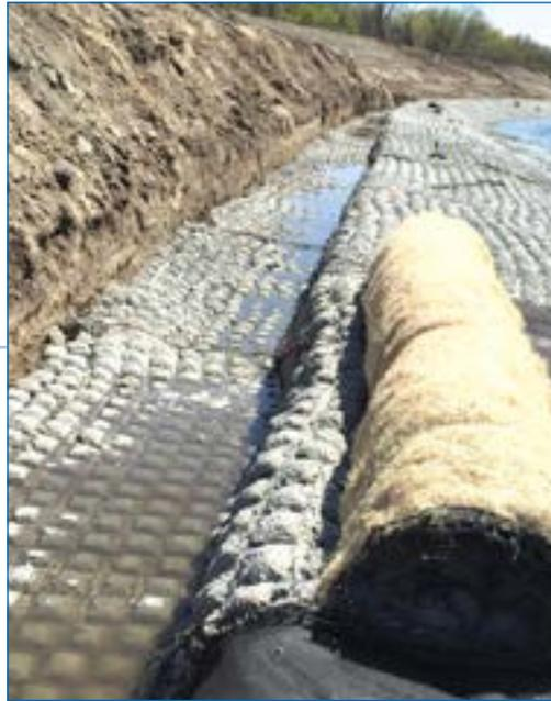
4 Flexamat in the anchor trench and ready to be deployed into the water.
