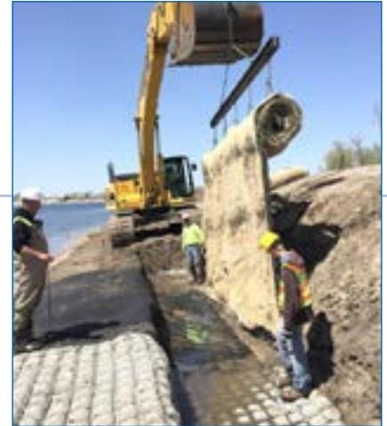
5 Simple equipment can be used to install Flexamat.
