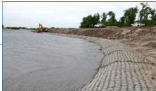
7 Flexamat is installed quickly.
