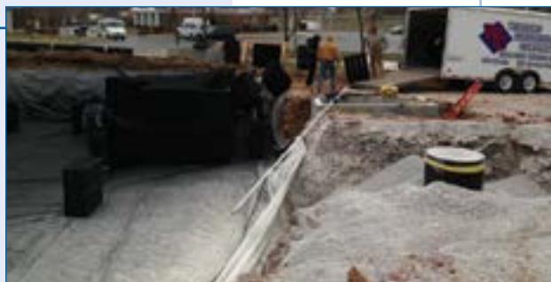
3 Duquesne project using preassembled Raintanks.
