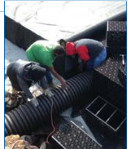
5 Connecting inflow pipe from the water quality unit.
