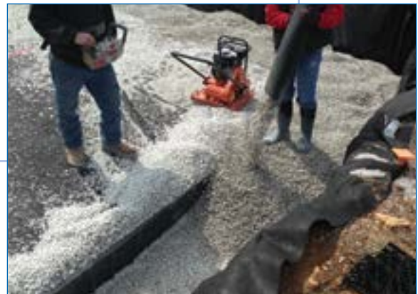
6 Backfilling and compacting the aggregate.
