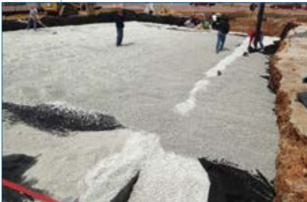
7 Completed detention system preparing for pavement.
