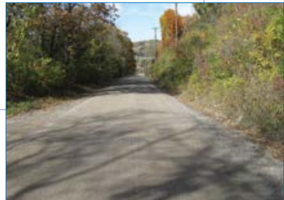
6 Before CSO work.
