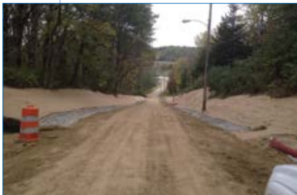
7 Both ditches after work.
