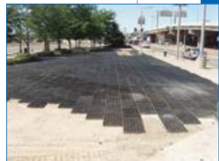
2 70% of the Geoblock 5150 is installed.
