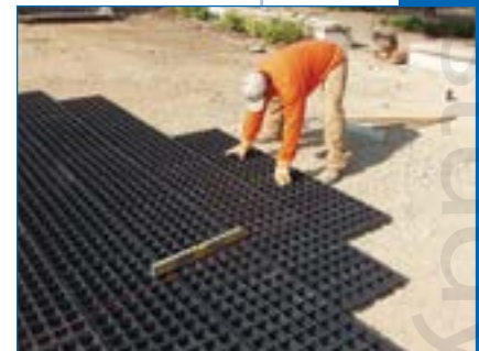
1 The Herringbone pattern was utilized here.
