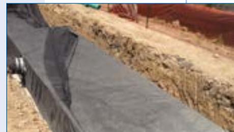
3 A 1 foot space is minimum on the sides with compacted rock placed for stability.
