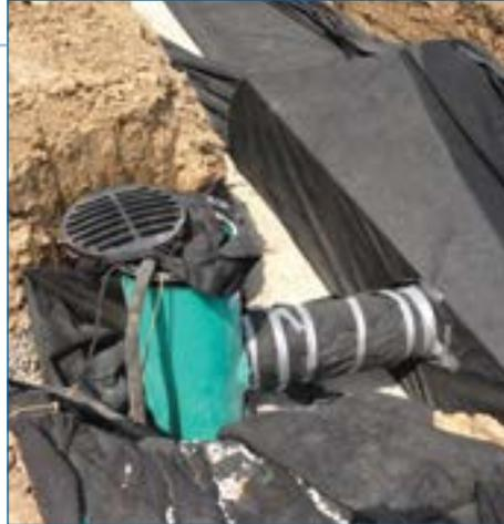
**4** The Nyloplast Drain Basin is connected to the tanks with pipe.
