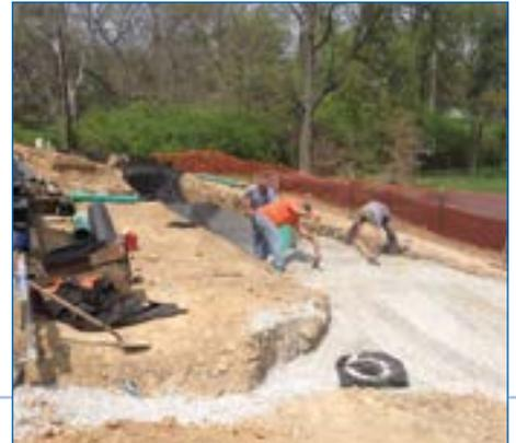
**6** Continuing to place the rock backfill.
