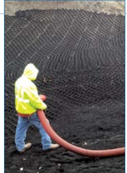
4 Amended soils introduced in the cells.
