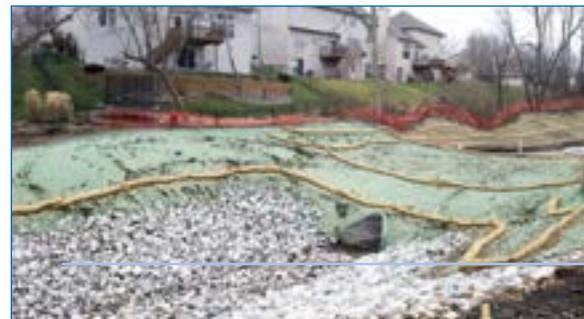
5 Flexterra mulch and seeded.
