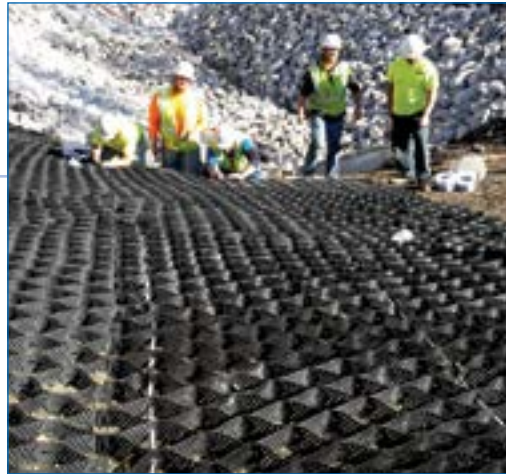
3 Note the support tendons distributing the load evenly through the section.
