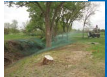
1 Installation rate of 3500 lbs/acre.
