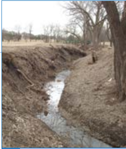
4 Creek before installation.
