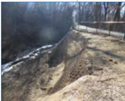
6 Completed Wall before Spring.
