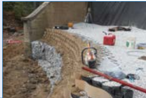
2 Geoweb wall construction on top of the Gabion Base.
