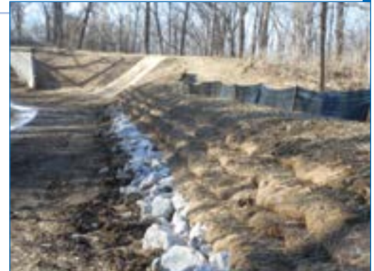
5 Completed project before vegetation growth.
