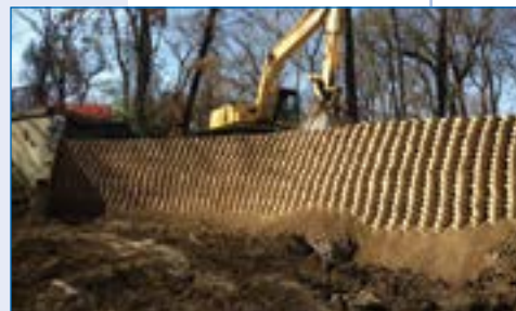
3 Geoweb wall supporting track hoe during infill.
