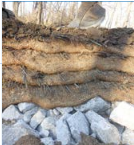
4 "Burrito Wall" during construction.
