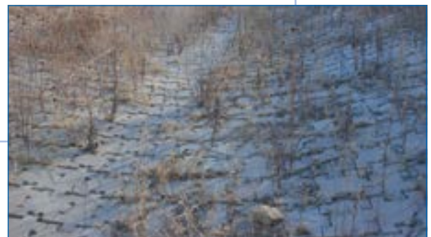
7 The channel 4 years later, no problems!
