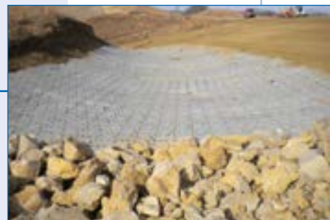
3 Upstream toe protection.
