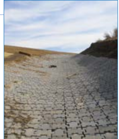
5 Looking upstream from the midway point.
