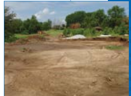
1 Dirt work beginning May 2014.
