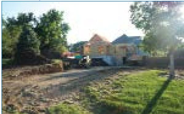
**6** Site under construction with new addition framing and side yard excavating to create walkout.
