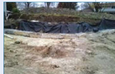
2 Wall construction with aggregate footing, 4oz nonwoven filter fabric and drainage rock.
