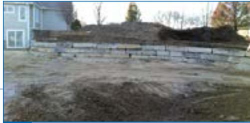
**3** Completed north lower terraced wall (approx. 84 tons used).
